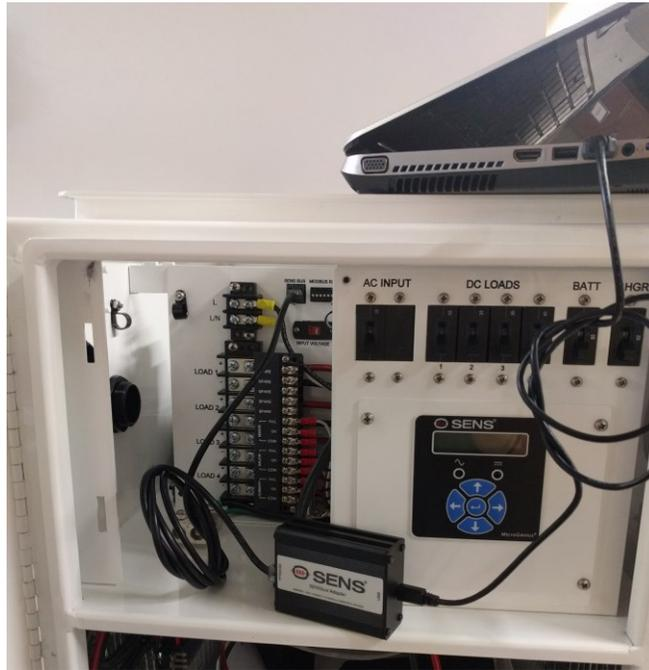
6.4.3. Optional TCP/IP Modbus and SENSbus USB Communications Wiring
