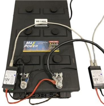
One of the two sensors is then connected to one of the ports on the rear of the SC4 Site Controller in the Genset BMS cabinet. The Genset BMS ships with a 25-foot CAT5 cable (PBT-PAC-CAT5-25) spooled inside the cabinet for each battery string connected to the SC4.
